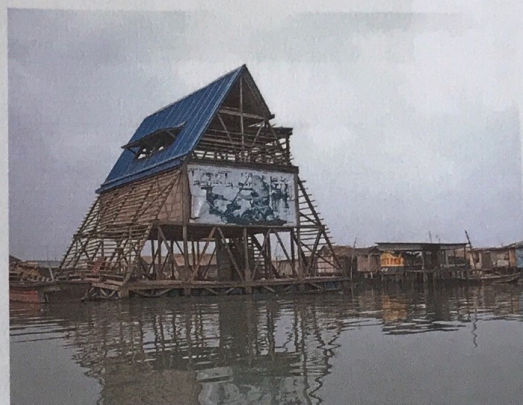
The Makoko Floating School stood tall above the surrounding houses before it collapsed.
